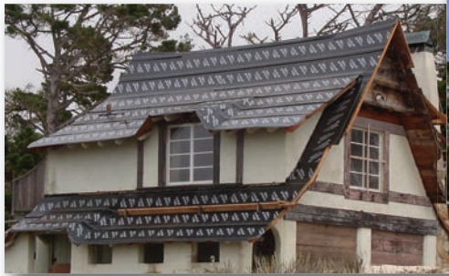
Waterproof roofing paper was applied
