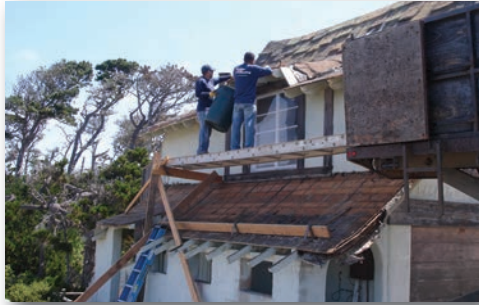
Eleven tons of concrete tiles were removed from the roof
