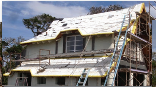
Each tile was replaced with the same size lightweight foam material
