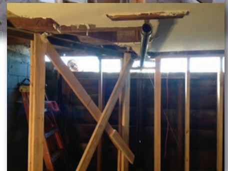
Much of the interior work is yet to be completed
